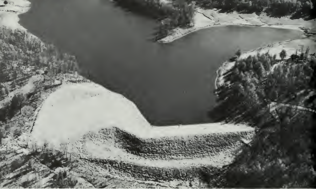
A floodwater-retarding structure on Six Mile Creek.
